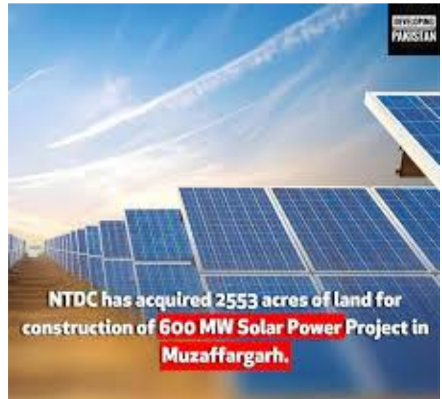
Figure 4. Muzaffargarh solar project [37]
